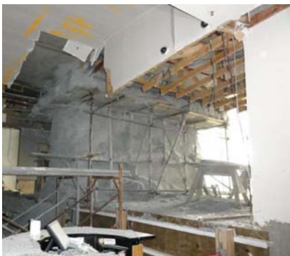
Overall View of Repair Using Shotcrete
